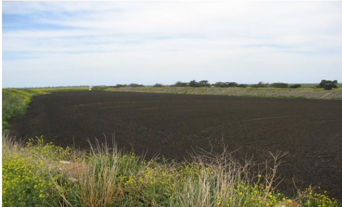
Sludge Storage Lagoon
