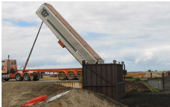
Truck delivering biosolids at Sludge Storage Lagoons
