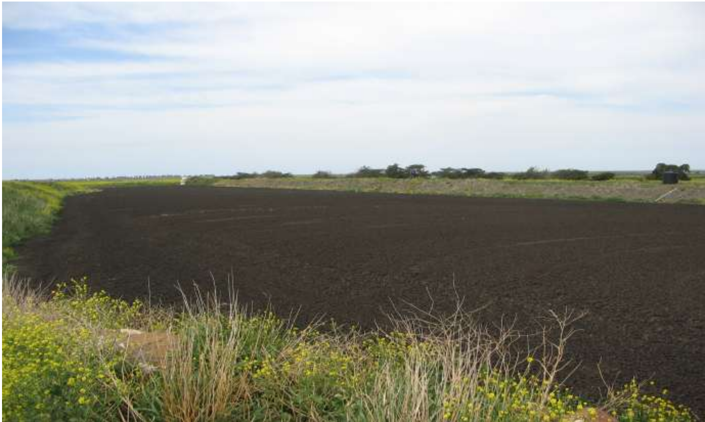
Sludge Storage Lagoon
