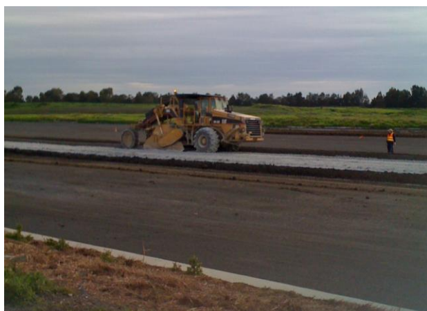
Figure 1: Blending of lime with biosolids
