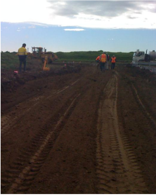
Figure 2: Cement/lime amended biosolids placed in road
