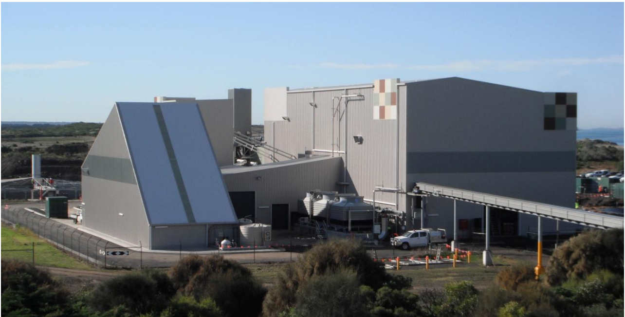
Figure 1 - View of Biosolids Plant from the Black Rock Water Reclamation Plant
