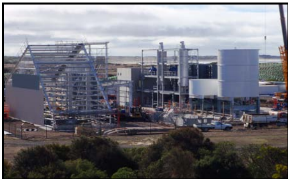
Construction of Black Rock Water Reclamation Plant
