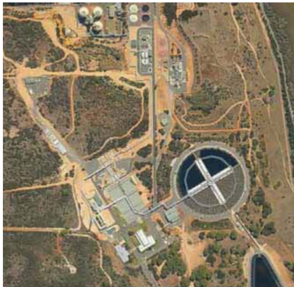
Figure 1. An aerial view of Woodman Point WWTP, Perth, Western Australia.
