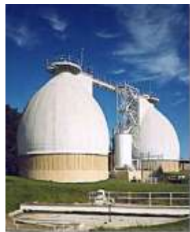
Anaerobic Digesters
