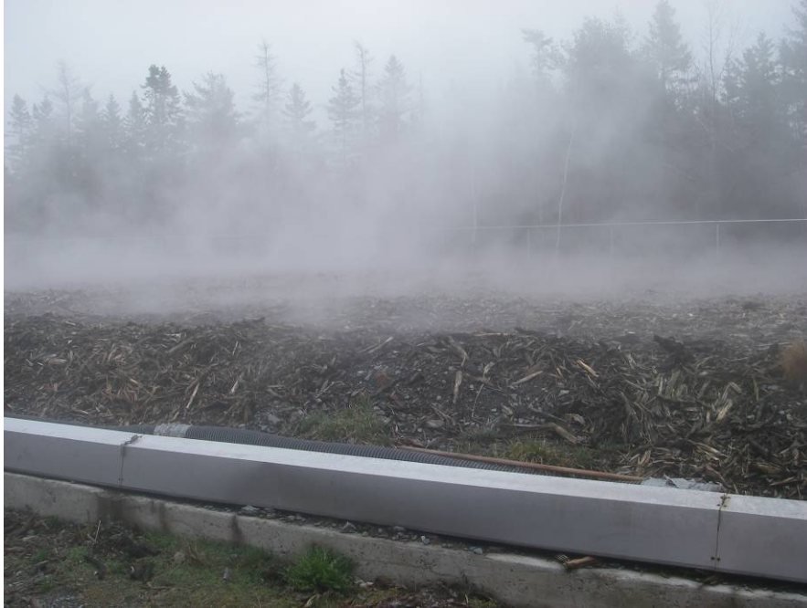
Figure 6. Surface of Biofilter for Process Air Treatment
