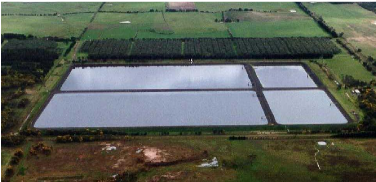
Figure 1 – Aerial View of Typical Facultative Lagoon
