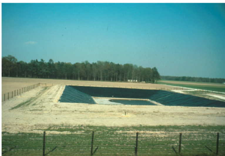
Figure 3.1 A lined lagoon (US EPA/USDA, 2000)
